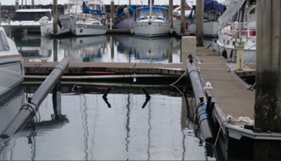
Above: From the water this is what you have got to aim at. Tolerances driving a catamaran are much tighter than with a mono-hull. Twin motors mounted wide are an assistance but approach to an Airberth in a cat are far from lassaize faire . Below: This picture is complementary to that of the Airberth ready to receive a vessel. As the knuckle of the bows come onto the forward crossbeam, small ramps (not seen) provide for a smooth arrival on top of the crossbeam and the angle guides do the job for lateral centring. It is still pretty easy, just not as easy as the promo DVD infers.
